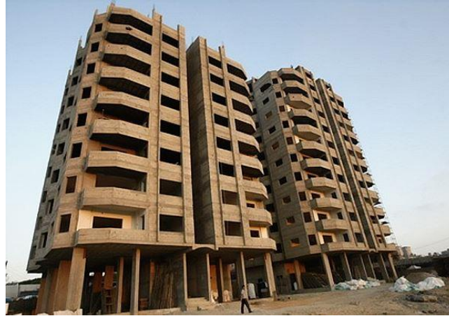
Fig. (3.5): Building Frame System.
