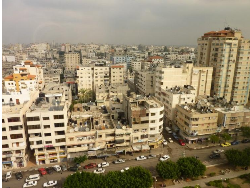
Fig. (3.2): Reinforced Concrete Buildings in Gaza.
