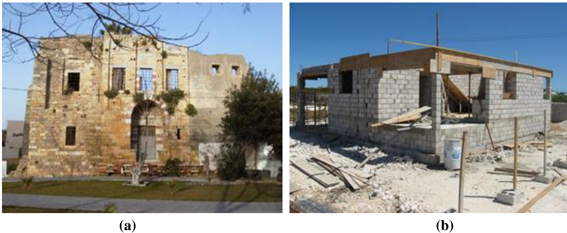
Fig. (3.1): Unreinforced Masonry Buildings, (a) Concrete block building, (b) Sand stone building.
