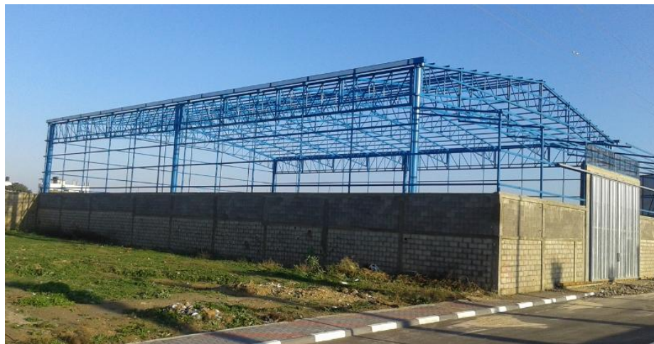
Fig. (3.3): Steel Structure in Gaza Strip.
