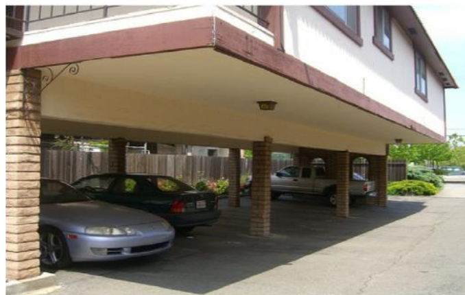
Fig. (3.7): Building with Cantilever Slab.
